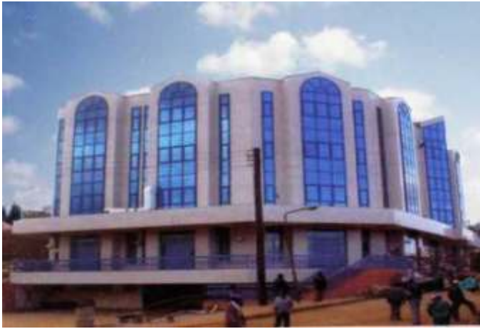
Mwalimu Co-operative Plaza. Completed in 2003
